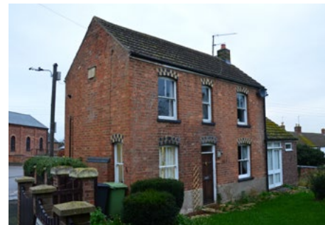
Decorative use of polychromatic brickwork 54 South Street
