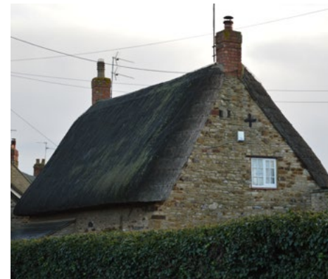
12 Church Street with traditional long straw thatch
